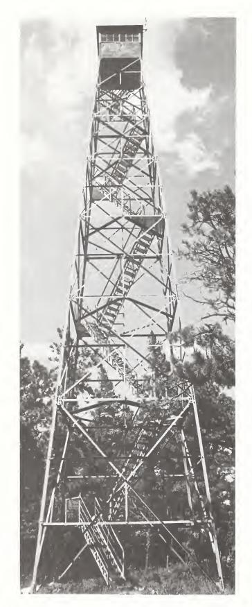
Figure 218. Carrisa lookout, an Aermotor MC-39 with an 80 feet high steel tower, built in 1934.
